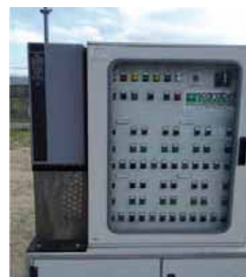
Inverter Danfoss VLT Aqua Drive FC 202 in IP66
